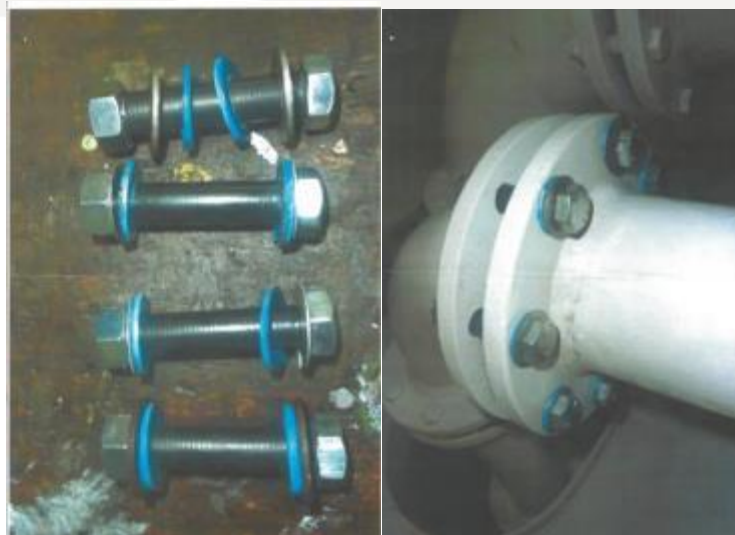
Flange and screws insulation
